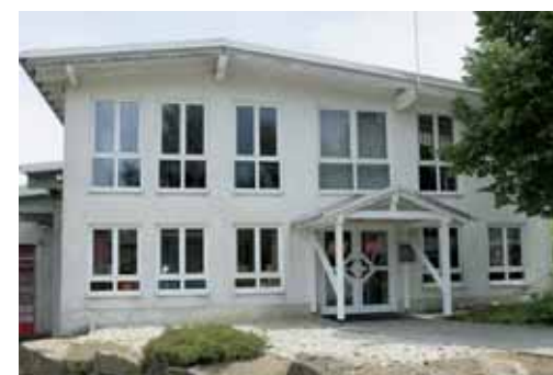
AVE HEAD OFFICE AT THE LOCATION OF INNERZELL-HILGENREITH IN BAVARIA
