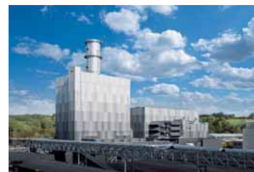
THE COMBINED-CYCLE GAS TURBINE POWER PLANT IS THE BIGGEST ENERGY-EFFICIENCY MEASURE IN THE HISTORY OF UPPER AUSTRIA. CO 2 EMISSIONS PER GENERATED KILOWATT HOUR ARE REDUCED BY 66 PER CENT AND NO x EMISSIONS BY ALMOST 90 PER CENT.
